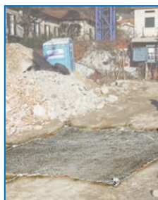
Stendere accuratamente la rete Carefully spread the net
